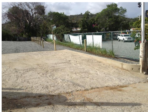
Figure 46. Gravel filter and parking lot stabilization by PDC in Parguera, Puerto Rico.
