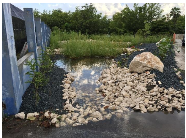
Figure 42. BMPs implemented following a train treatment approach in Yauco, Puerto Rico. Practices include bioswales, bioretentions and raingardens.
