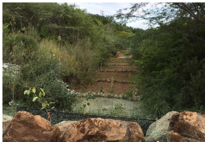
Figure 41. BMPs implemented following a train treatment approach in Puerto del Manglar in Culebra, Puerto Rico. Practices include bioswales and sediment traps.
