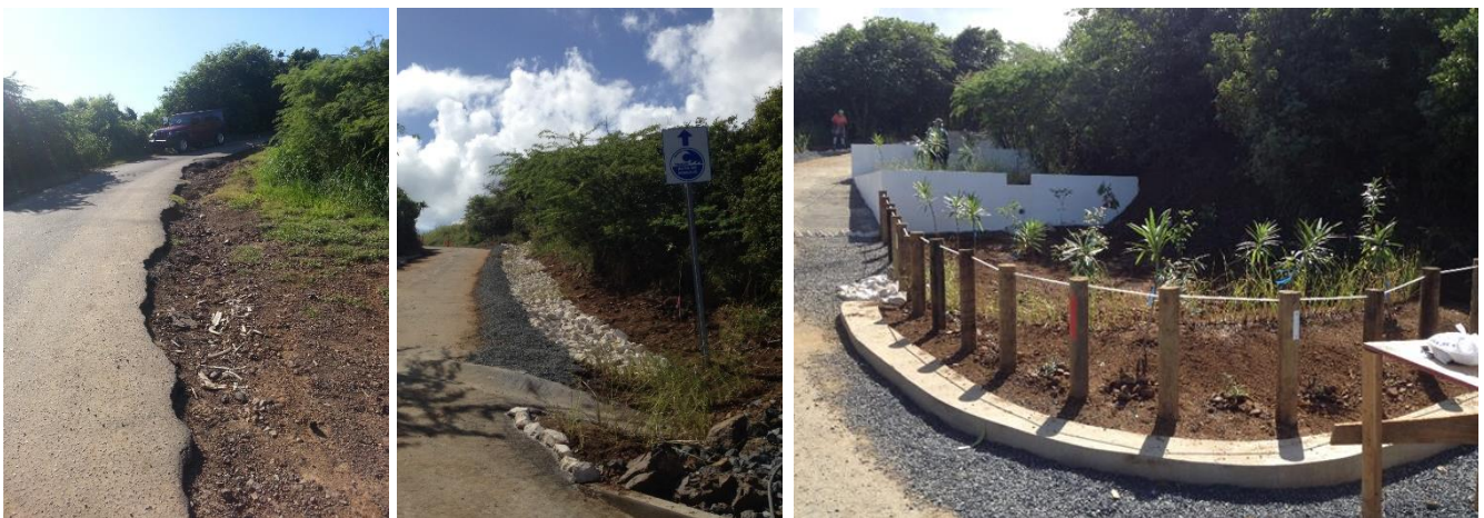
Figure 38. BMPs implemented following a train treatment approach in Zoni Beach at Culebra Puerto Rico. Practices include bioswales, bioretentions, raingardens and permeable parking.
