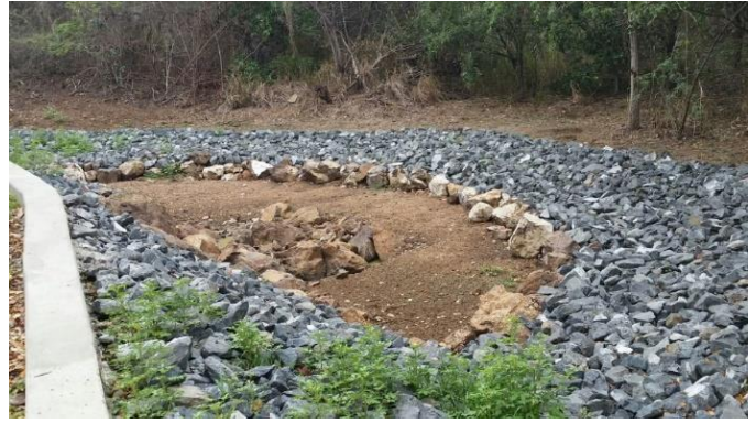
Figure 39. BMPs implemented following a train treatment approach in Punta Soldado in Culebra, Puerto Rico. Practices include bioswales, bioretentions, raingardens, sediment traps and permeable parking.
