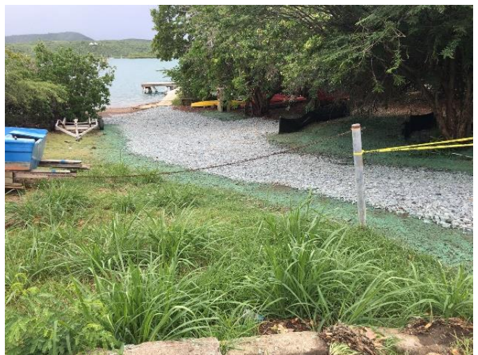
Figure 40. BMPs implemented following a train treatment approach in Fulladosa Culebra, Puerto Rico. Practices include bioswales and raingardens.
