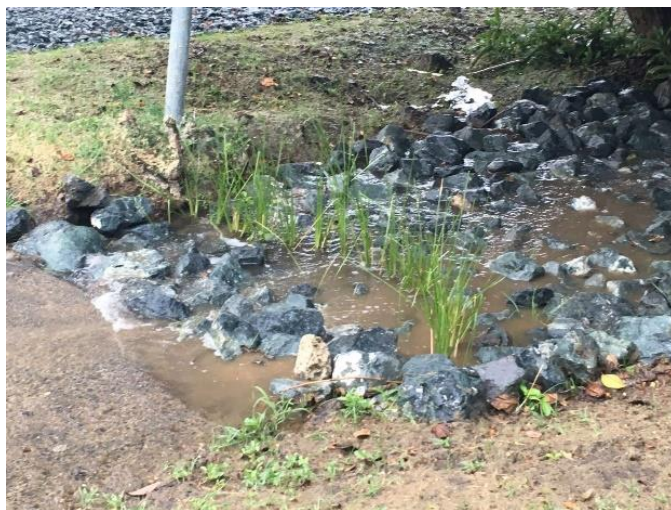
Figure 40. BMPs implemented following a train treatment approach in Fulladosa Culebra, Puerto Rico. Practices include bioswales and raingardens.
