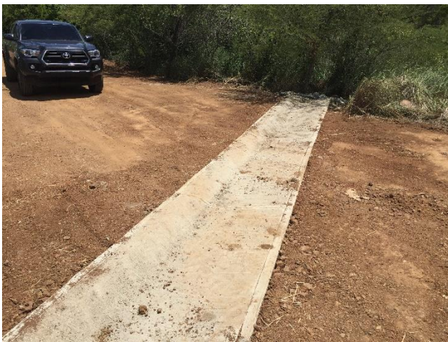
Figure 59. Example of swales made by PDC in Culebra (concrete) and in a coffee farm (stones).
