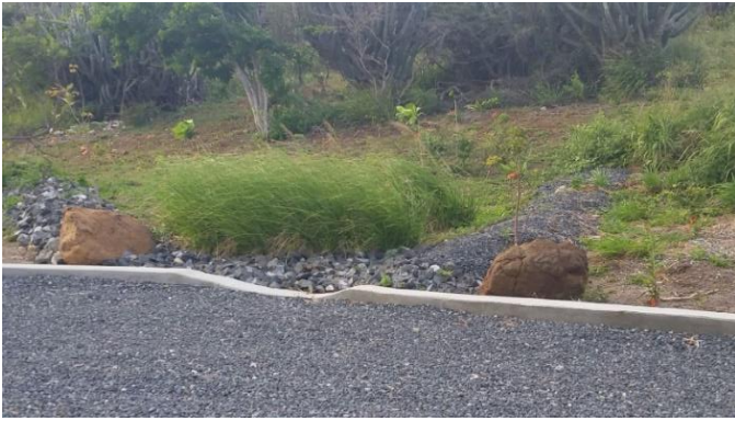
Figure 39. BMPs implemented following a train treatment approach in Punta Soldado in Culebra, Puerto Rico. Practices include bioswales, bioretentions, raingardens, sediment traps and permeable parking.
