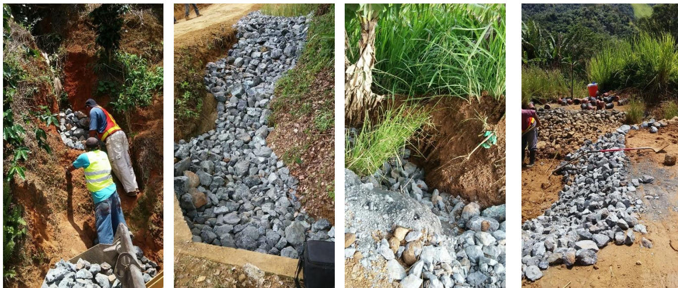
Figure 57. Examples of rip-rap practices implemented by PDC on a coffee Farm on Yauco Puerto Rico.
