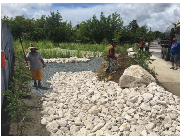
Figure 42. BMPs implemented following a train treatment approach in Yauco, Puerto Rico. Practices include bioswales, bioretentions and raingardens.
