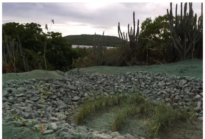
Figure 41. BMPs implemented following a train treatment approach in Puerto del Manglar in Culebra, Puerto Rico. Practices include bioswales and sediment traps.
