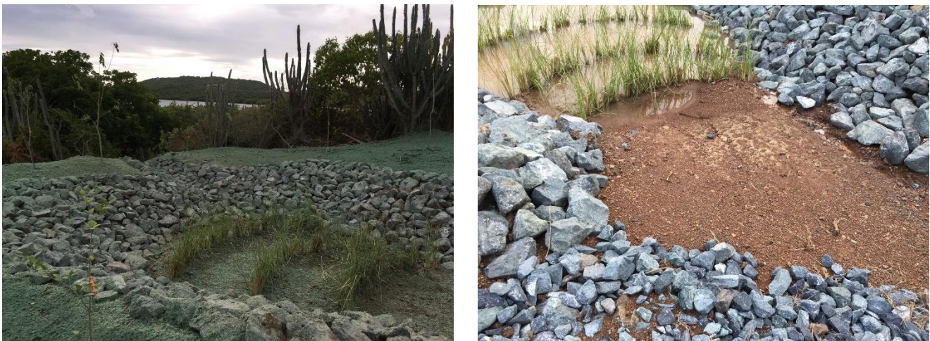
Figure 55. Example of a sediment trap built by PDC in Culebra Puerto Rico.
