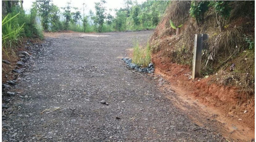
Figure 56. Example of gavel pavement done by PDC on a coffee farm on Yauco Puerto Rico
